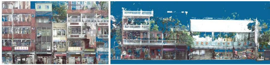
Fig. 7. The old street facade with different characteristics
