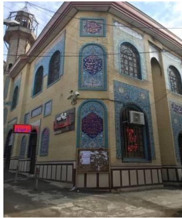
Figure 10 External Building Façade of the Shafei Mosque
