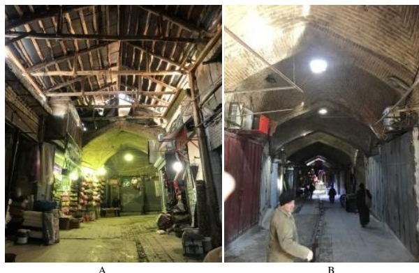
Figure 11 Tarikeh Bazaar (Dark Market) (A) Indoor Façade ; and (B) Another Side of Bazar
