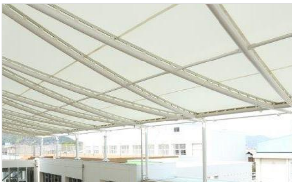
Fig. 15. Kagawa prefecture Sanuki City Shido elementary school, Kagawa, Japan
