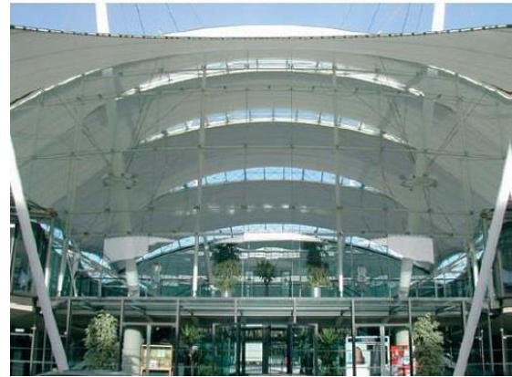
Fig. 20. Operable windows on perimeter glazed walls, Inland Revenue Amenity building, Nottingham, UK (Michael Hopkins Partners, 1995)
