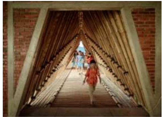
Fig. 2. School of Alfa Omega/RAW Architecture: Use of bamboo and bricks for sustainable buildings
