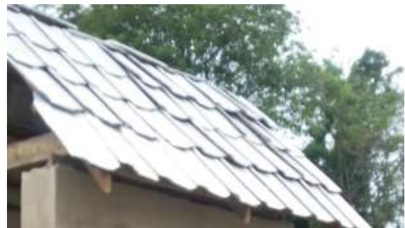
Fig. 10. KF/CCA/Cement Roof tiles demonstration
