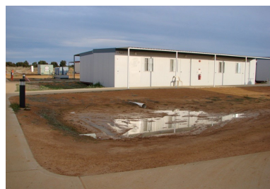
Plates 4 and 5. Poor Drainage
