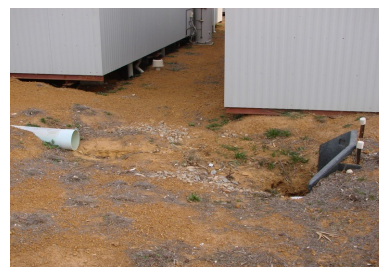
Plates 4 and 5. Poor Drainage
